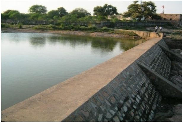
Atmaram Water harvesting structure, Hatideh
