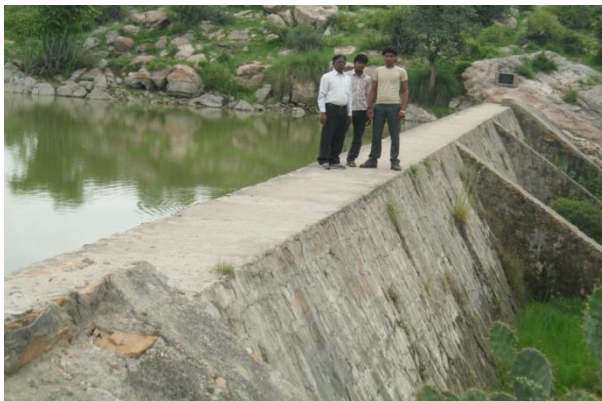
Johadwala Water harvesting structure, Loharabas
